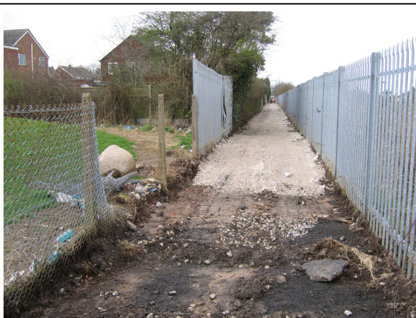
Malpas Road to Heath Road Greenway: during construction.
