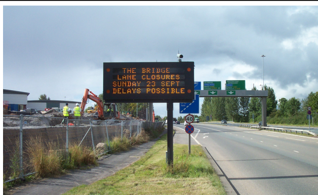
VMS with ANPR camera, Bridgewater Expressway
